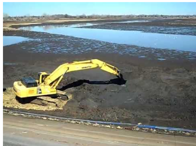
Fig 1.5 Slit removal from River bed
