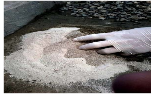
Fig.1 Glass Powder Being Mixed With Sand
