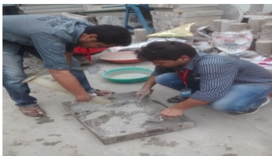
Fig 1. Mixing of concrete
