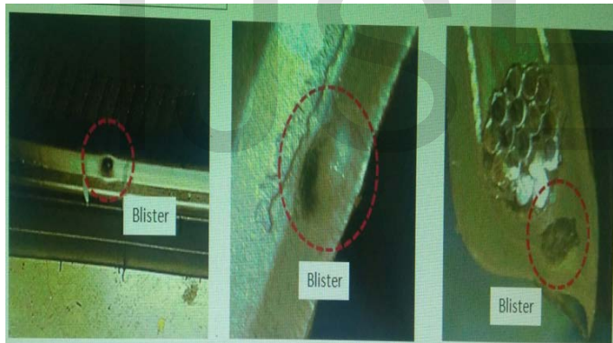
Figure 3. Visual defect blistered bead base.
